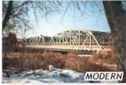
The "Green" bridge
