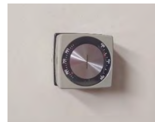
Typical Pneumatic Thermostat
