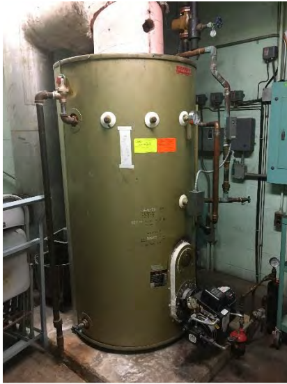
Oil fired water heater
