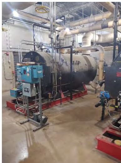
Heating Hot Water Boilers
